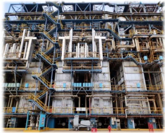
Figure 1. External structure of ethylene cracking furnace.
